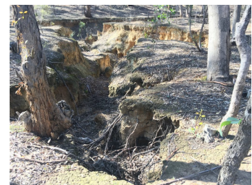
Badly eroded gully, Photo by Paul Foreman
